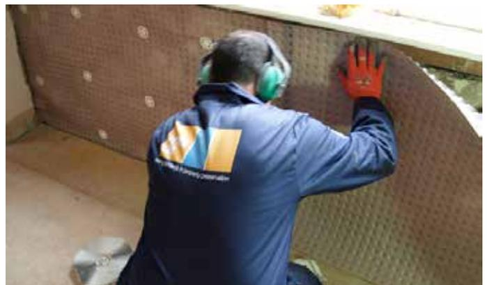
lapped and sealed. It involves adequately disposing of water, either by gravity, or through a sump and pump to a suitable outlet. This must be designed with adequate access points for servicing and maintenance, and a one-way valve to prevent backflow.
