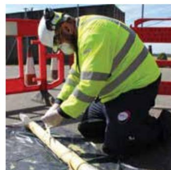
The company has been among the first to use lining to strengthen highway drains as part of smart motorway modernisation programme, and to use UV lining to rehabilitate industrial pipes that need chemical resistance.
